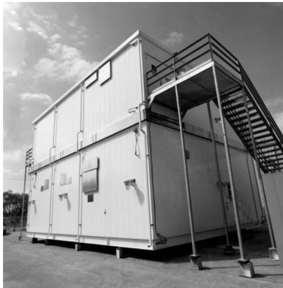
Two Story Integrated Power Assembly
